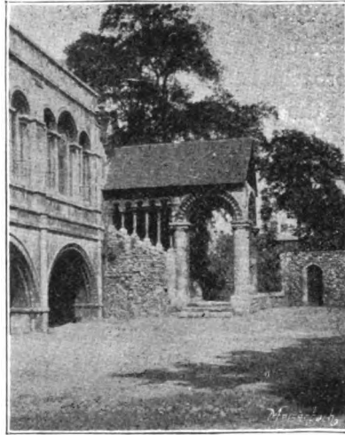
Norman Staircase, Canterbury Cathedral.
