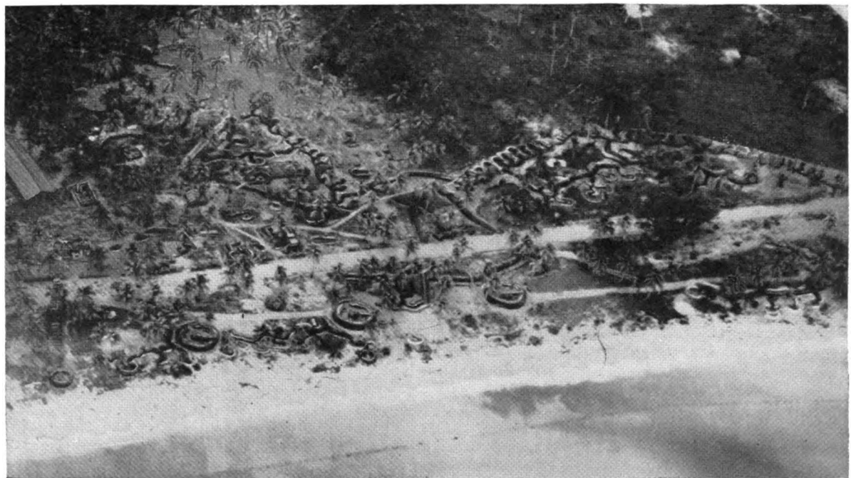
Figure 113. A typical coastal defense strongpoint.
