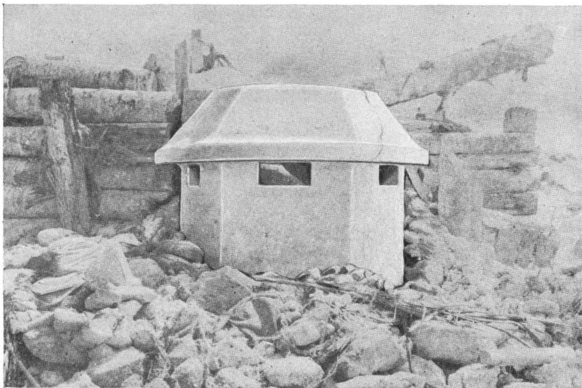
Figure 146. A concrete pillbox.
