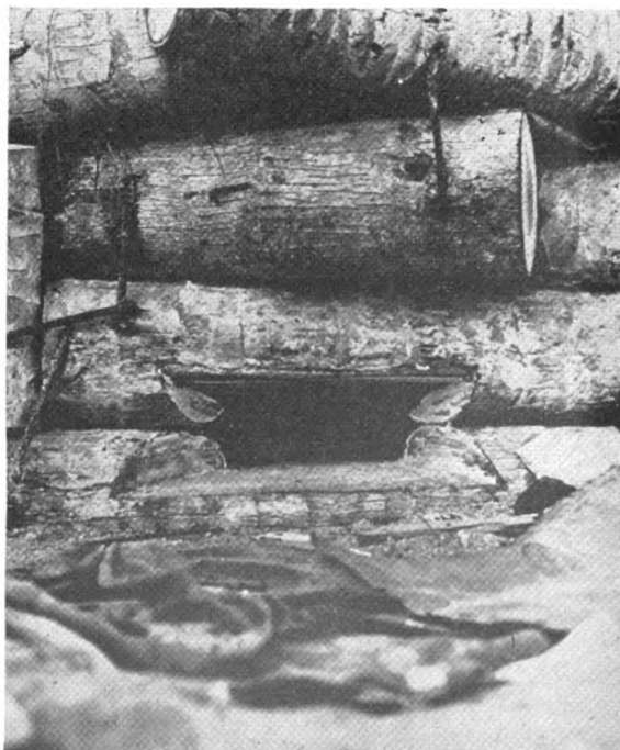
Figure 141. Front view of a pillbox.
