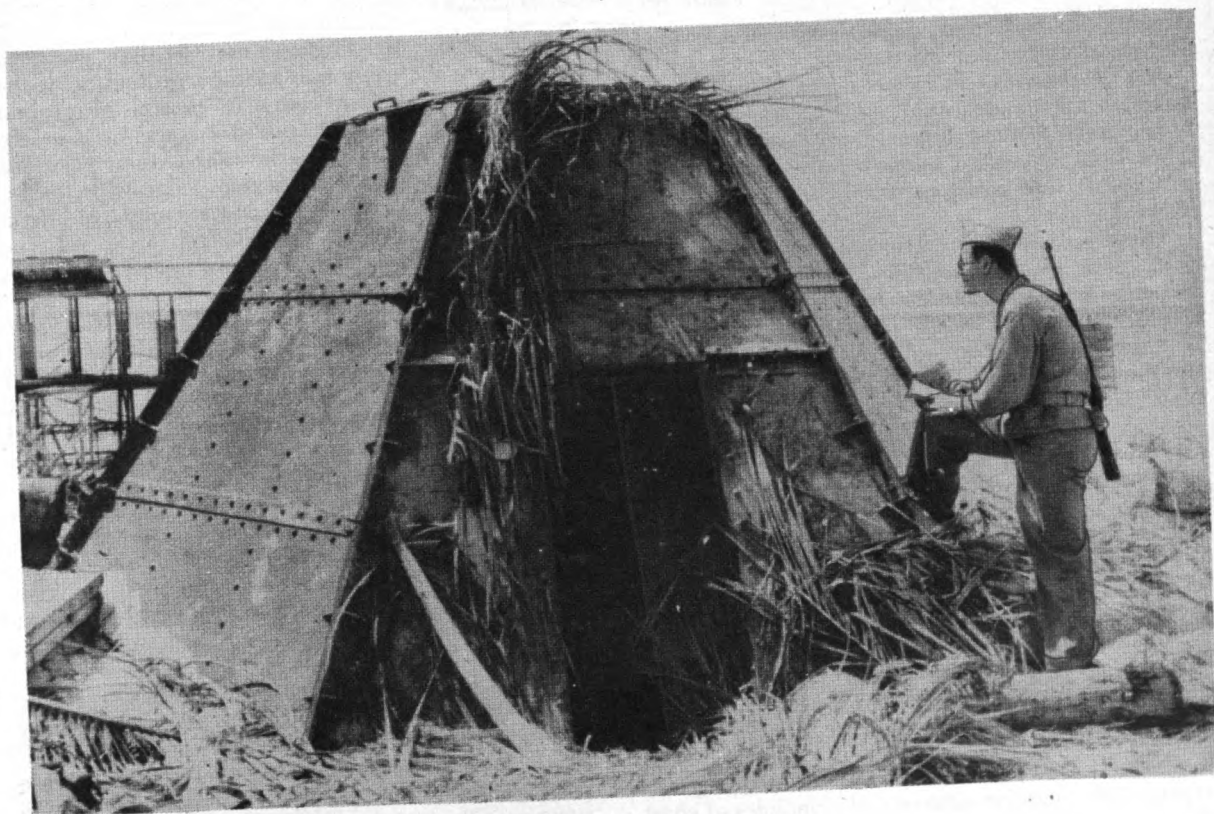
Figure 145. A hexagonal steel pillbox.
