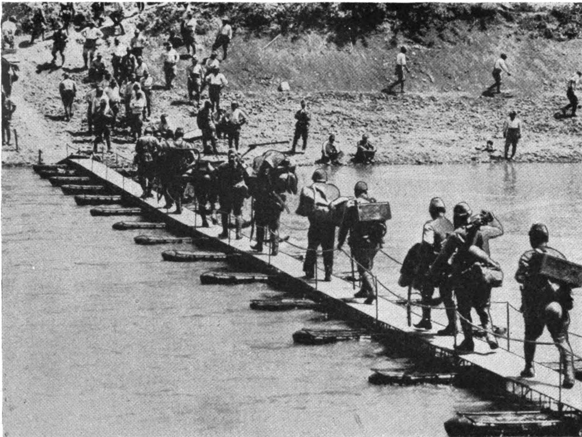
Figure 380. Small ponton bridge.
