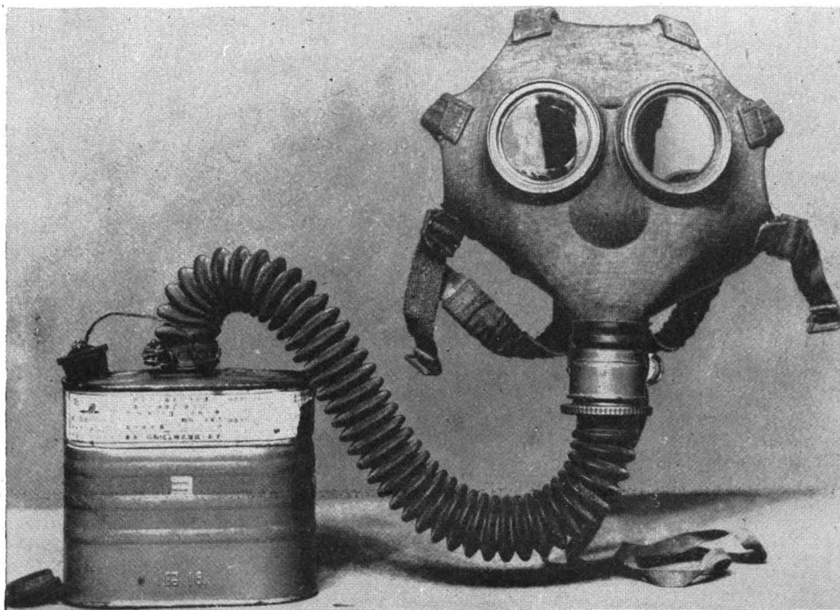
Figure 260. Civilian gas mask type 1, model A (Improved).
