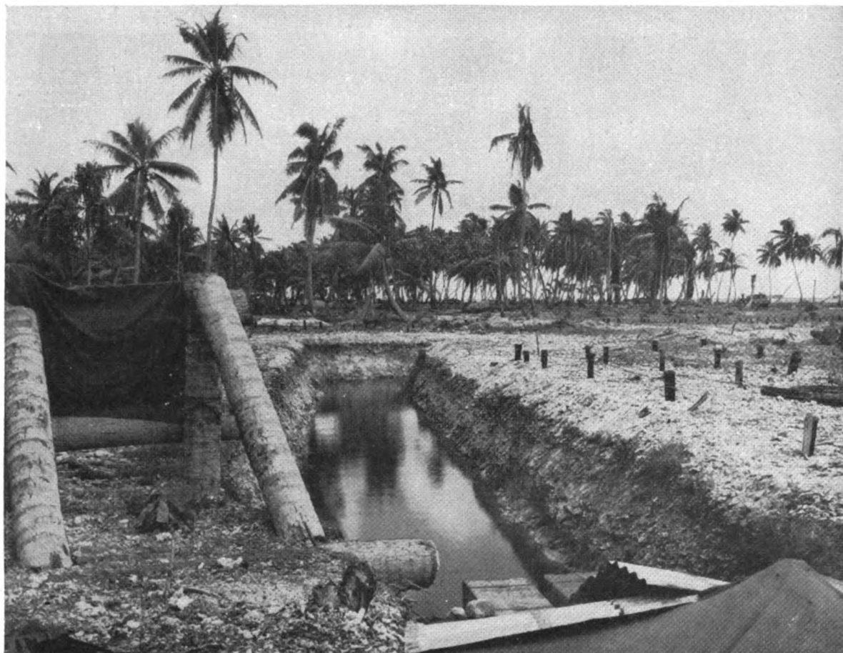
Figure 114. Antitank ditch.
