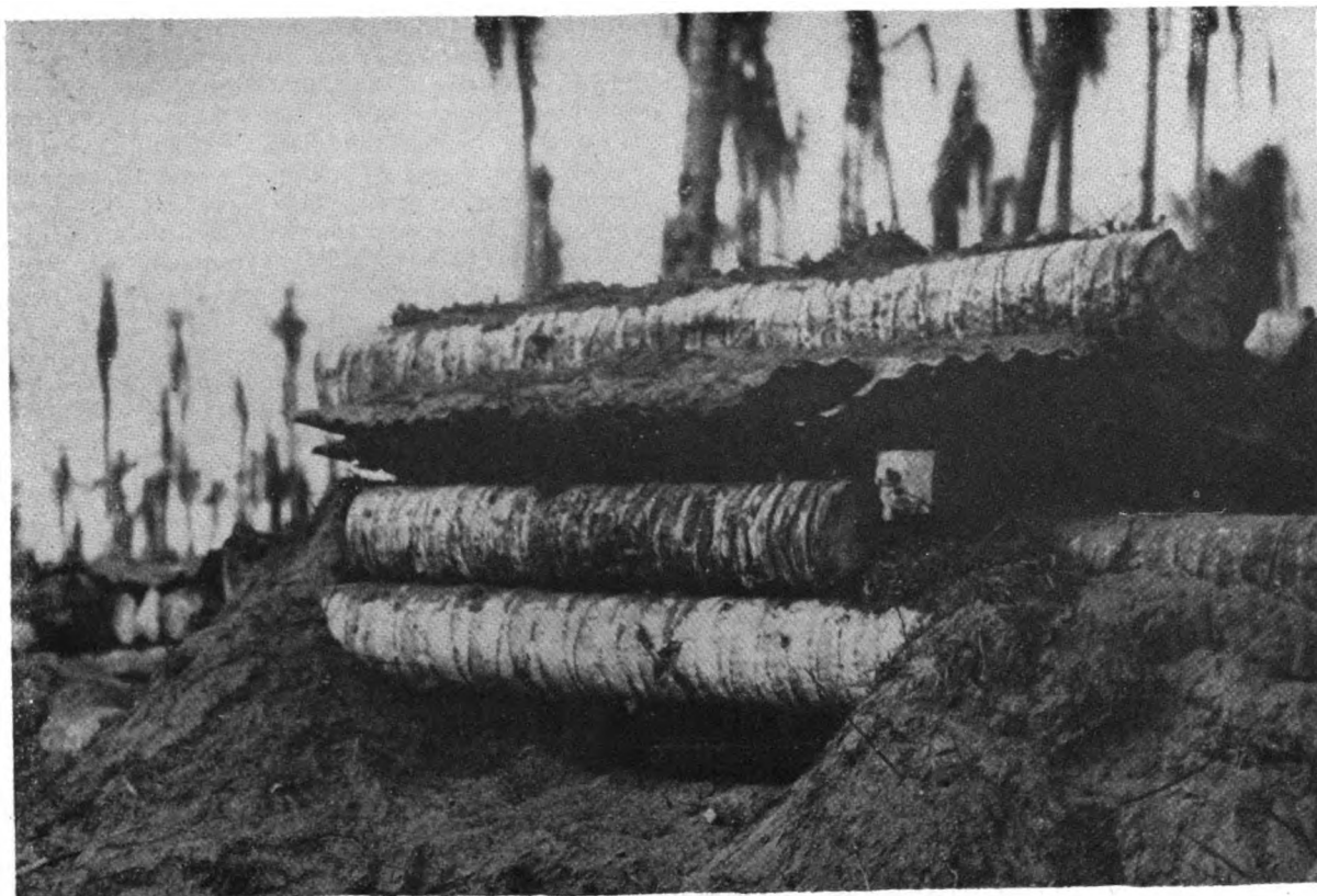
Figure 143. Exterior view of pillbox.
